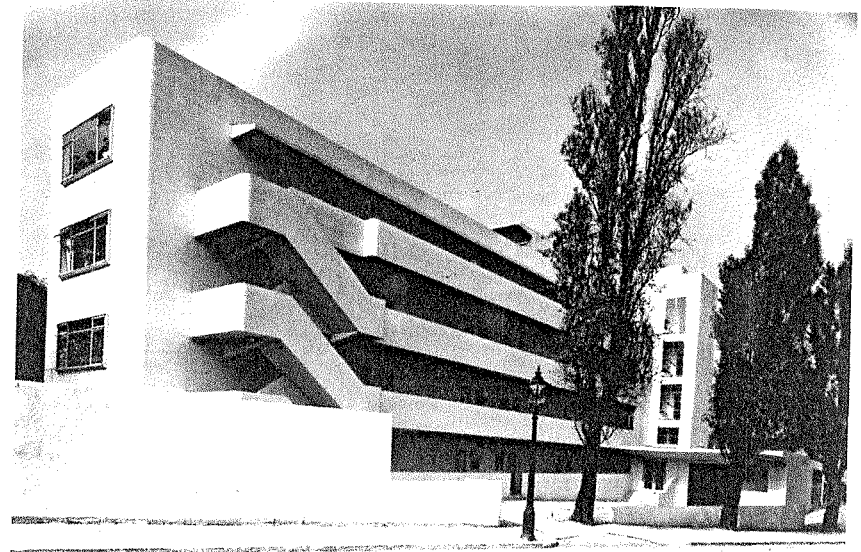
Figure 9.5. Wells Coates, Lawn Road Flats, Hampstead, London, 1934 (Architectural Press Archive / RIBA Collections, RIBA2508-9).
