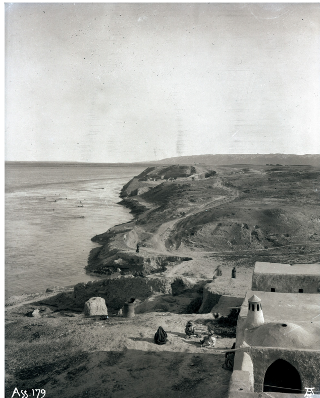
Fig. B2.6: A view from the rooftop of the expedition house across the southern appended buildings, taken on 2 April 1904. Ass Ph 179 (© SMB, VAM, DOG; photo by Walter Andrae).
