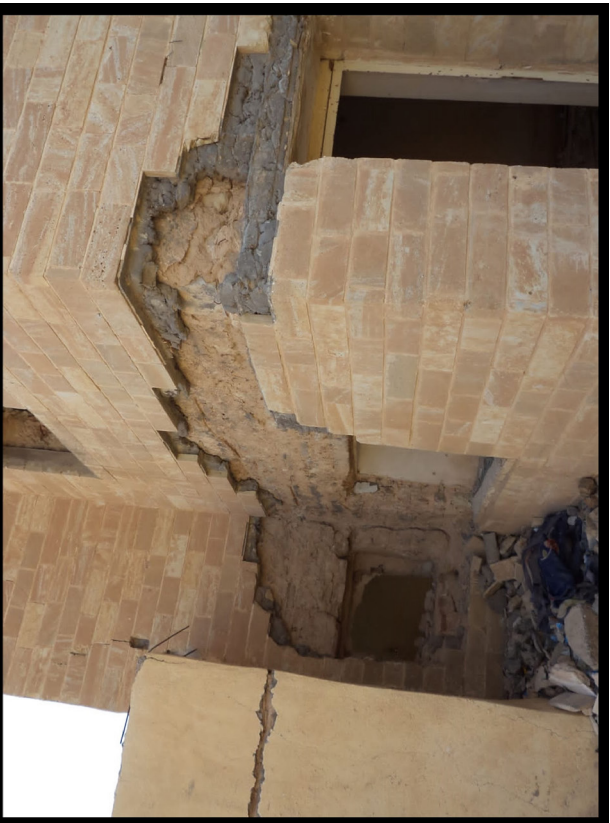
Fig. B1.6: The façade of the southeastern block of the excavation house, before and after restoration. Photos by Akam Omar Ahmed Al-Qaradaghi.
