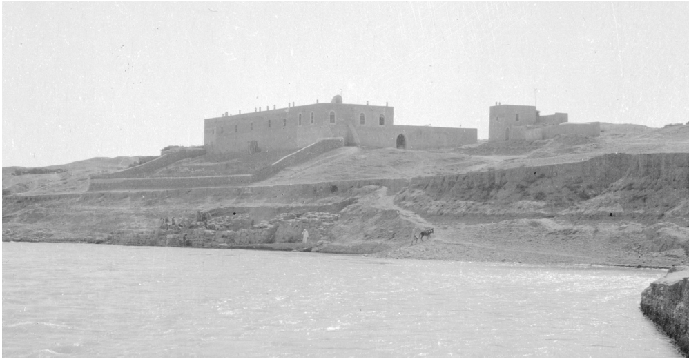
Fig. B2.25: The excavation house as seen from the river bank on 6 October 1904, looking southwest. Detail of Ass Ph 291 (© SMB, VAM, DOG; photo by Walter Andrae).
