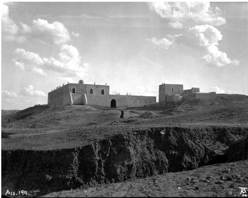
Fig. B2.18: View of the expedition house and Shaul Selman's house from the northeast, taken on 11 May 1904. Ass Ph 199 (© SMB, VAM, DOG; photo by Walter Andrae).
