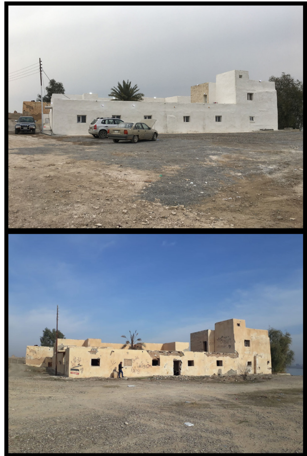
Fig. B1.1: The excavation house from the south, before and after restoration. Photos by Akam Omar Ahmed Al-Qaradaghi.
