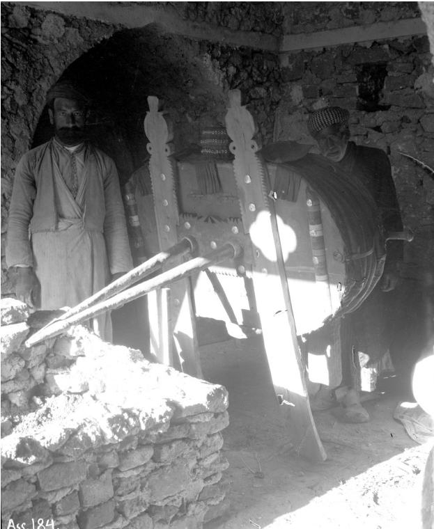
Fig. B2.12: View into the blacksmith workshop, during the construction of its forge on 11 May 1904. Ass Ph 184 (© SMB, VAM, DOG; photo by Walter Andrae).
