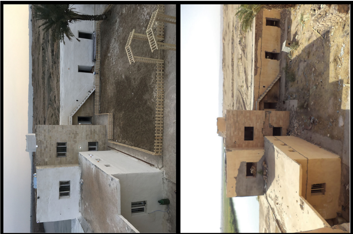
Fig. B1.10: The courtyard with the southern part of the east wing as seen from the roof of the north wing, before and after restoration. Photos by Akam Omar Ahmed Al-Qaradaghi.
