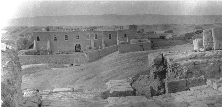
Fig. B2.21: The excavation house with front garden and surrounding buildings, looking south. Detail of a photo taken at some point after April 1912. Ass Ph 6184 (© SMB, VAM, DOG; photographer unknown).
