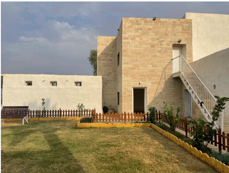
Fig. B4.4: View of the stone-lined façade of the southeastern corner of the excavation house as seen from the courtyard in November 2023. Photo by Andrea Squitieri.
