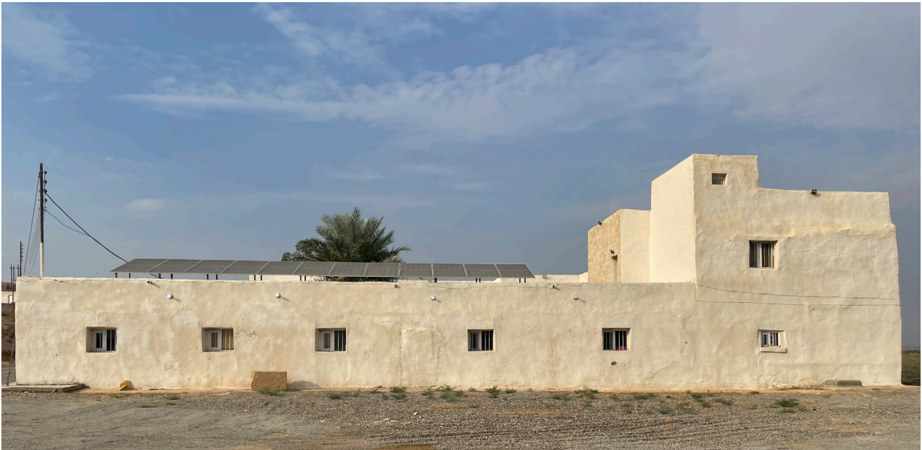
Fig. B5.4: View of the south wing of the excavation house, with the closed-up door visible in the centre of the façade. Photo by Andrea Squitieri.
