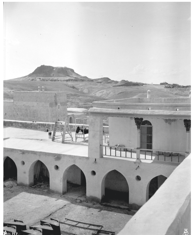
Fig. B2.16: View of the north wing of the expedition house on 11 May 1904, looking northwest across Shaul Selman's house towards the ziggurat of the Aššur temple. Ass Ph 197 (© SMB, VAM, DOG; photo by Walter Andrae).
