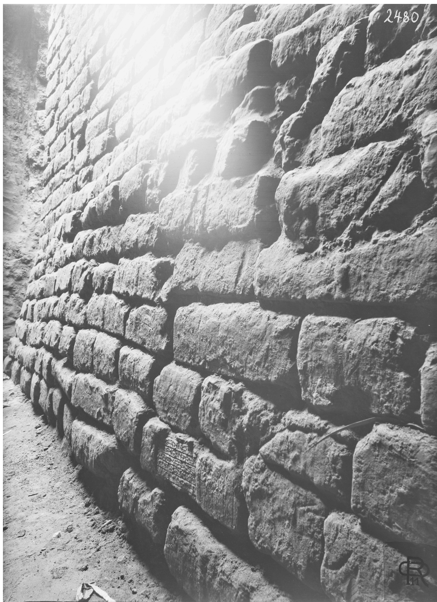
Figure 14. Bab ph 2480, which shows the embankment wall of the late channel (Kasr 2t) with an in-situ stamped brick (Npl. 11 ex. 7). © Staatliche Museen zu Berlin, Vorderasiatisches Museum, Deutsche Orient-Gesellschaft. Photo: Oscar Reuther, 1911.
