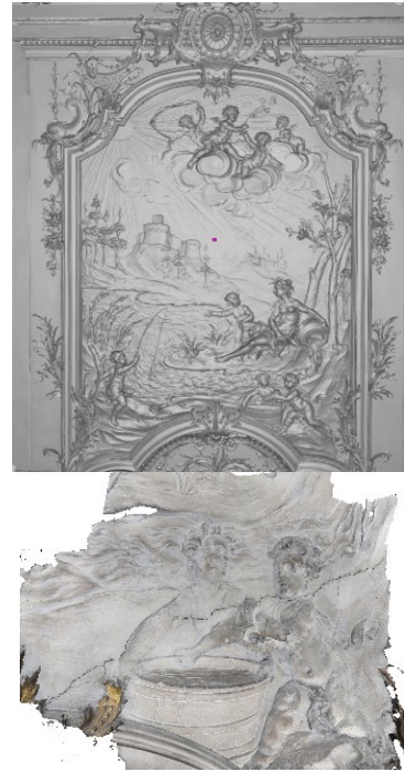
Figure 5. Supraporte stucco: top - untextured SL scan; bottom - photogrammetric model
