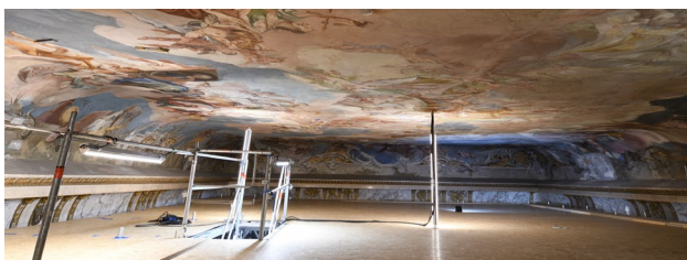
Figure 1. Ansbach ceiling with scaffolding platform
