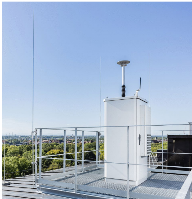
Fig. 2. Pollen monitor with required installations, © LGL, Alexander Harand.
