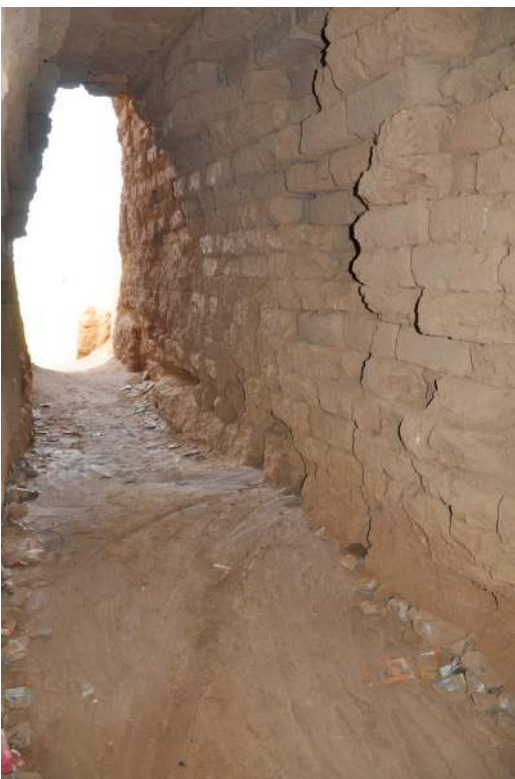
Fig. B1.6: The tunnel excavated in modern times within the ziggurat core. Photo by Eileen Eckmeier.
