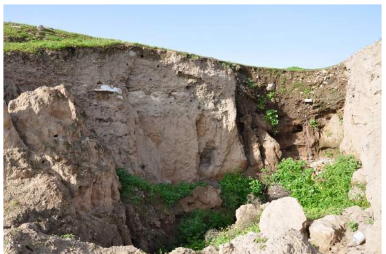
Fig. B1.9: Damage caused by rapid runoff during heavy rainfall. Photo by Eileen Eckmeier.
