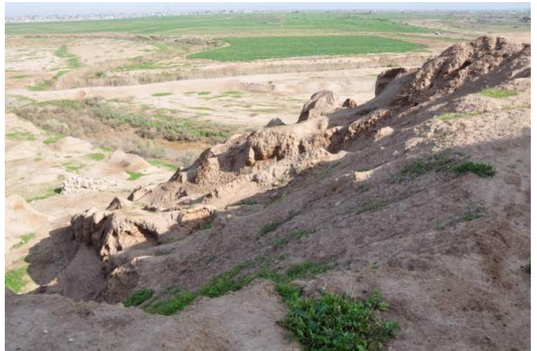
Fig. B1.8: Damage caused by slope erosion in the area below the ziggurat. Photo by Eileen Eckmeier.
