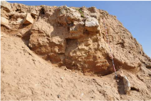
Fig. B1.18: Erosion along the city walls. Photo by Eileen Eckmeier.
