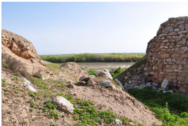
Fig. B1.11: Damage caused by rapid runoff during heavy rainfall. Photo by Eileen Eckmeier.
