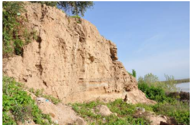
Fig. B1.22: Mudbrick structures cut by the river. Photo by Eileen Eckmeier.
