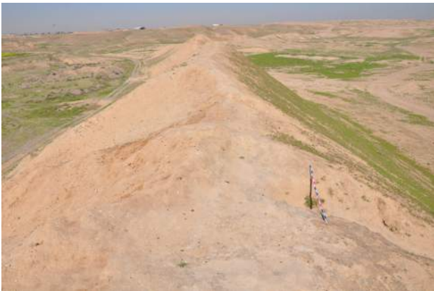
Fig. B1.19: Erosion along the city walls. Photo by Eileen Eckmeier.
