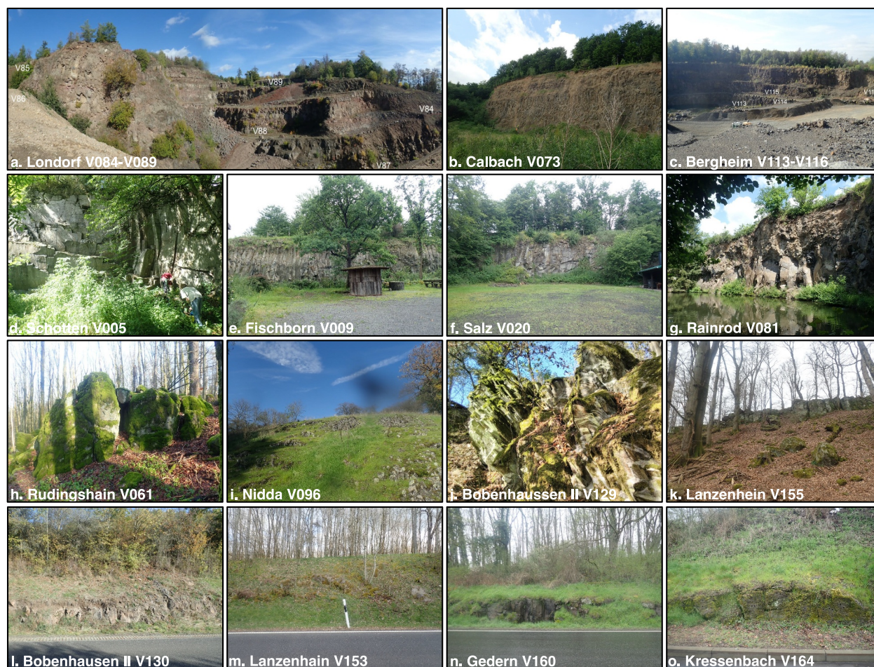
Figure 2. Field photographs of representative sites sampled from active quarries (a–c), previous quarries (d–g), natural outcrops (h–k), and road cuts (l–o).
