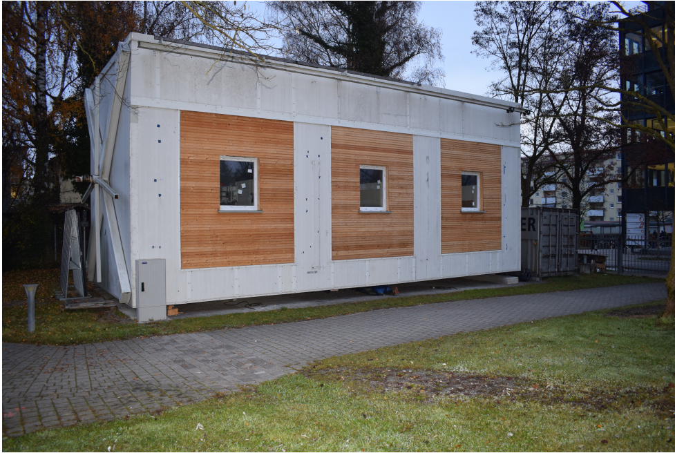
Figure 2.1: LiGT (= Labor für intelligente Gebäudetechnik = Laboratory for intelligent building technology) at the Technical University of Applied Sciences in Rosenheim.
