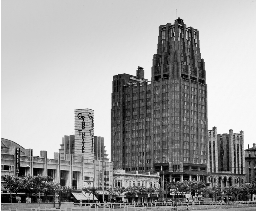
Fig. 6: Park Hotel and Grand Theatre Cinema in Shanghai. Architect L.E. Hudec 1931–1934 (Der Baumeister 1935).
