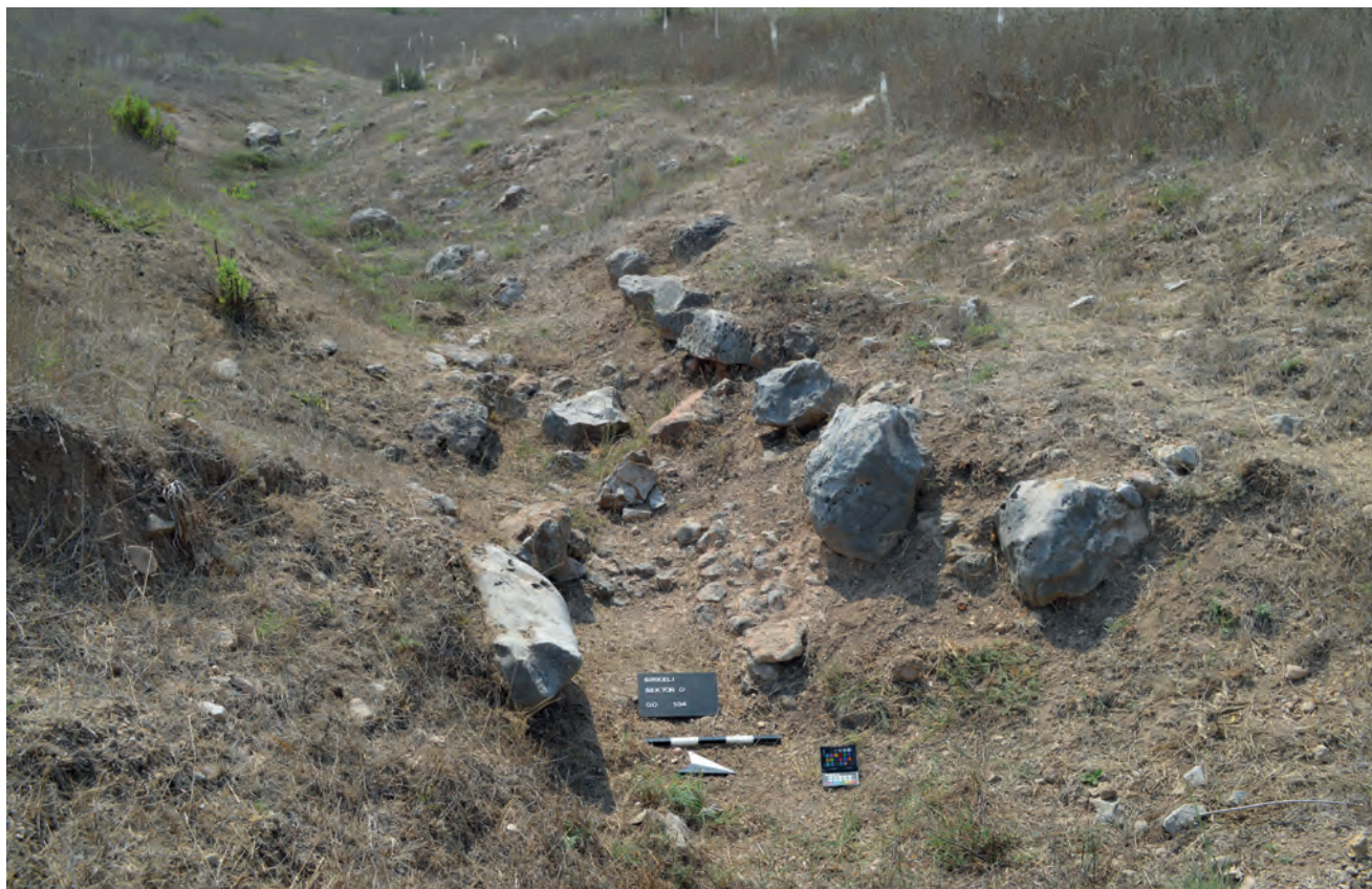
Fig. 4. Remains of the boundary walls of the channel in the Wadi south of Building O1 (Photo: A.E. Sollee).
