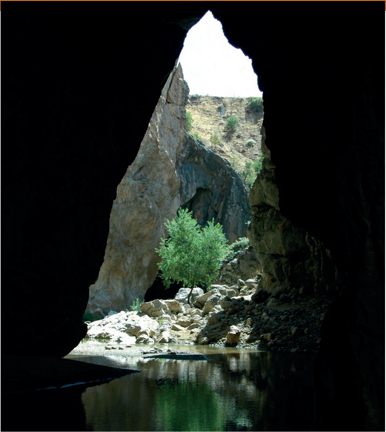
The entrance to the Tigris Tunnel, from the West – the collapsed last part of the river tunnel (Photo: A. Schachner).
