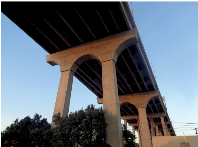
Figure 5: The Coronado Bridge.
